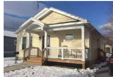
Division St. Habitat House
