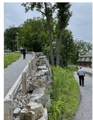
▲ Steep pedestrian pathway from Perimeter Road to Sussman Village Apartments
